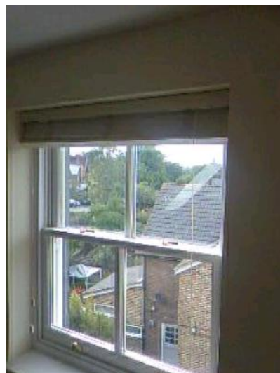
Lounge/Kitchen -Windows-Wooden Multi Pane, Double Glazed
