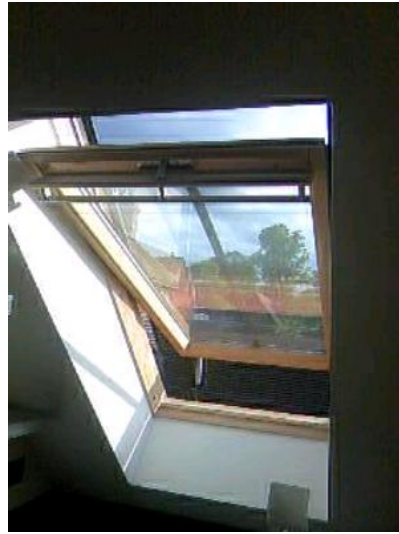
Lounge/Kitchen -Windows-Wooden Multi Pane, Double Glazed
