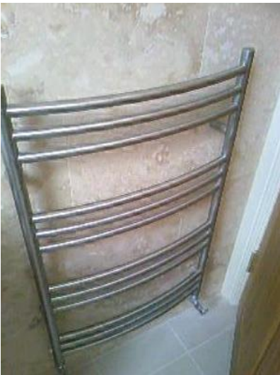
Bathroom-Heating-Wall Mounted Heated Towel Rail
