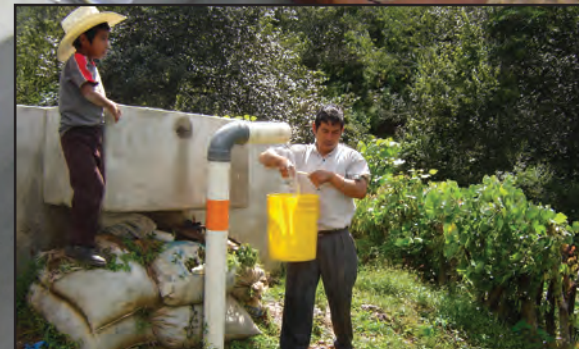
A filtering system eliminates most of the turbidity from the river water.
