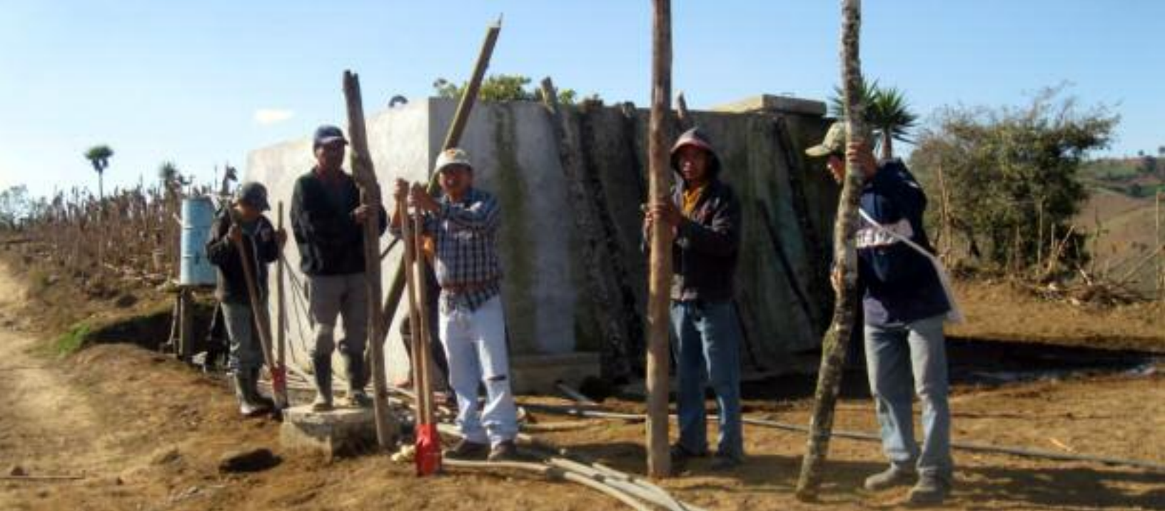
Thanks to funding from Oxfam, water systems damaged by Tropical Storm Agatha were repaired in nine communities.
